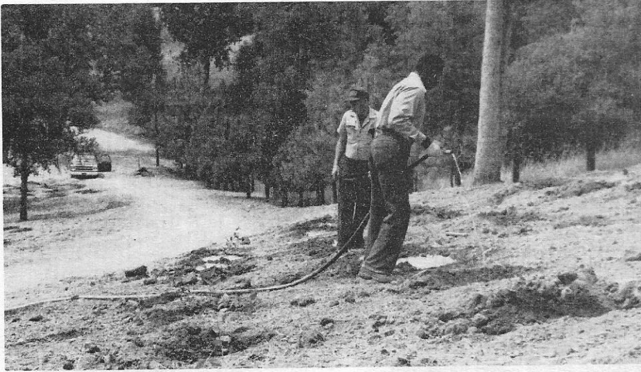
Fire crew supervisor Richard McAbee supervising installation of Fuel Wood Plantation Study Site at Miramonte Conservation Camp.
