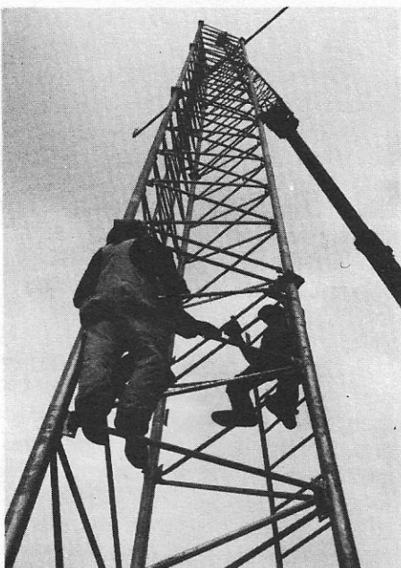
Workers guide the transmitter tower into proper location.
