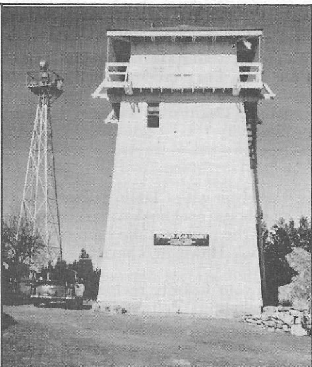
The Pacheco Peak lookout tower in Santa Clara County is a beautiful example of Dutch Windmill architecture and can be easily dismantled and moved to a new home. Anybody looking for a lookout??
