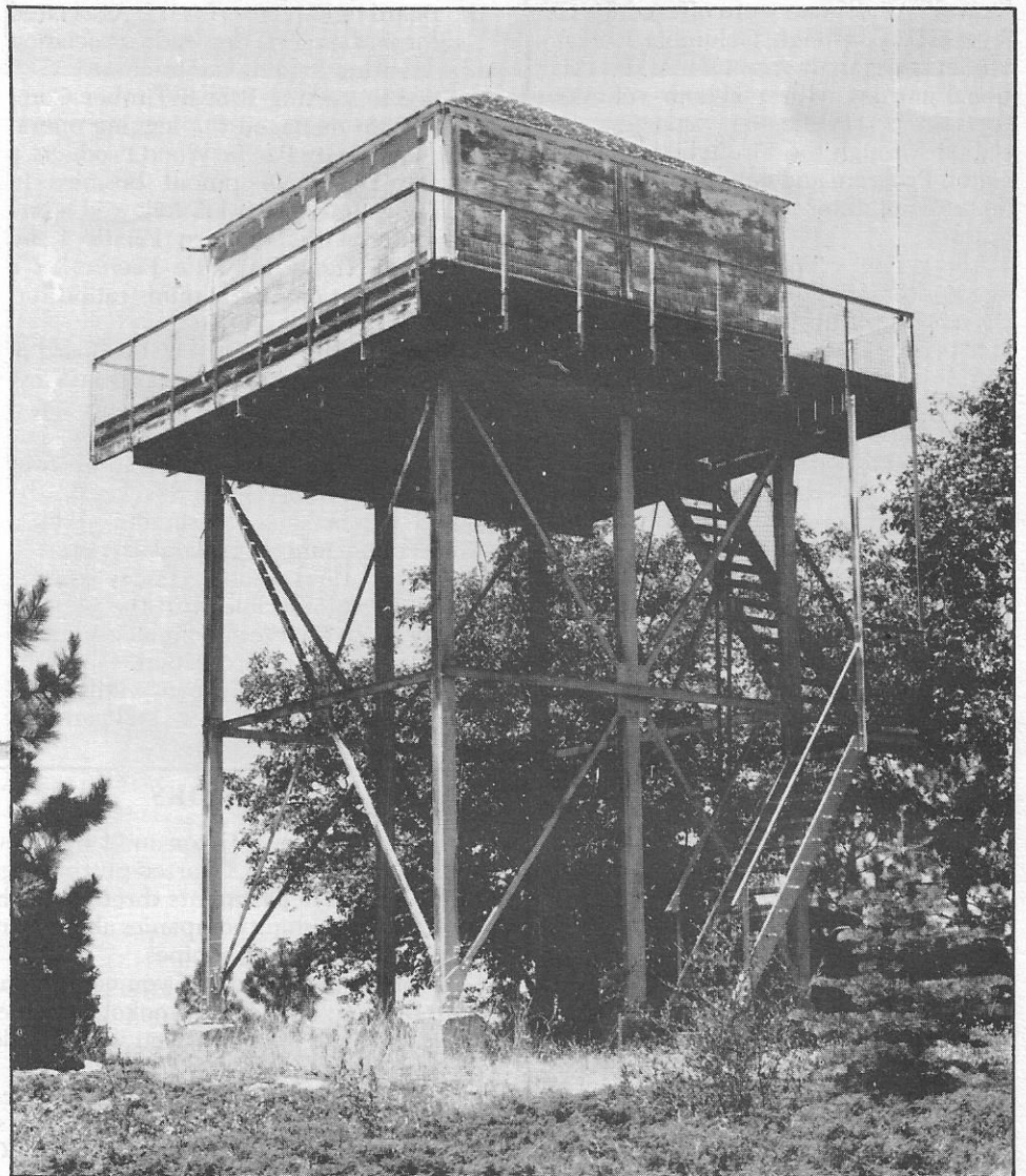
Following long and drawn out negotiations the Lookout Mountain tower will be moving to its new home at the El Dorado County Fairgrounds very soon.
