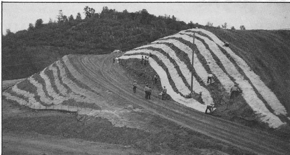
Erosion control work in Calaveras County.
