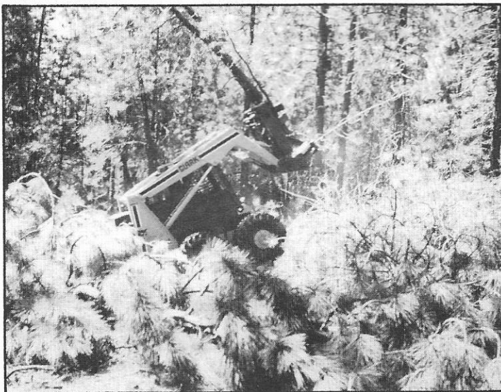
Here a feller-buncher is whipping a sheared off tree to a skidding pile.
