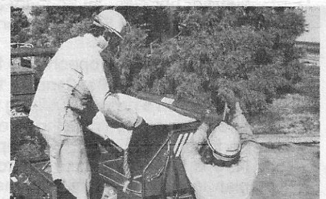
The blanket must be rolled in under the center "roller". The decal arrows should show the "underwound" direction of the roll.
